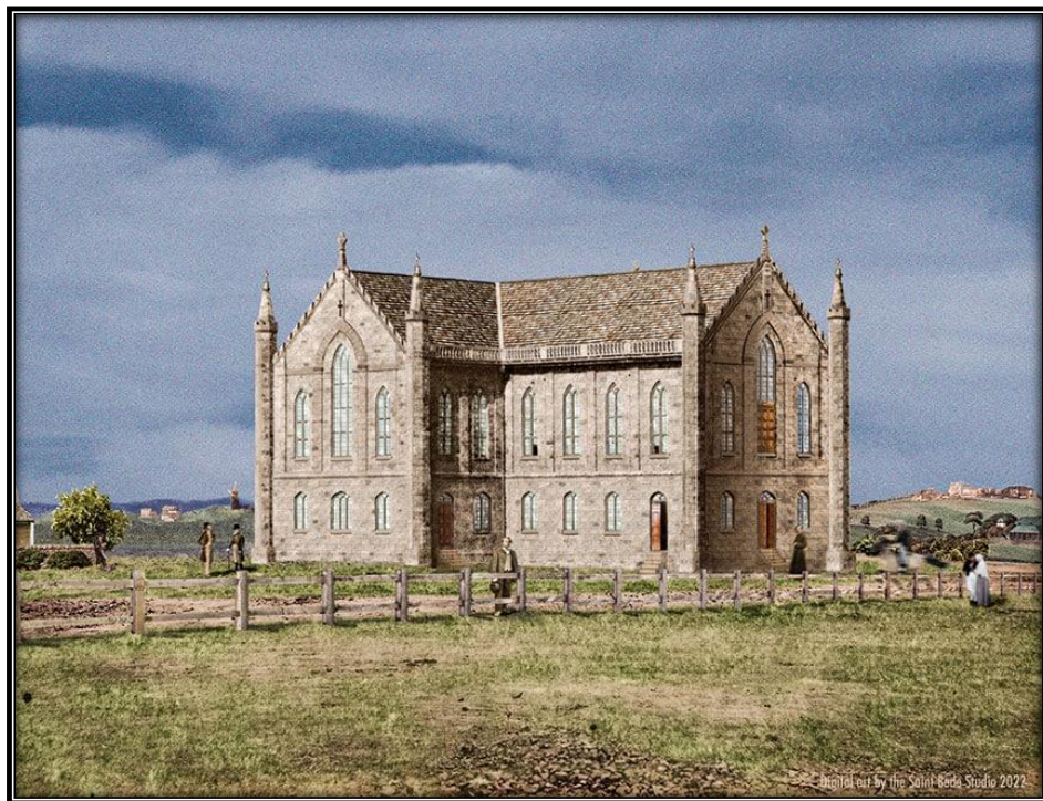
Initial work on the 'old' St Mary's Church began in 1822
